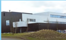
TRENKER LABORATORIES Nivelles, Belgium
